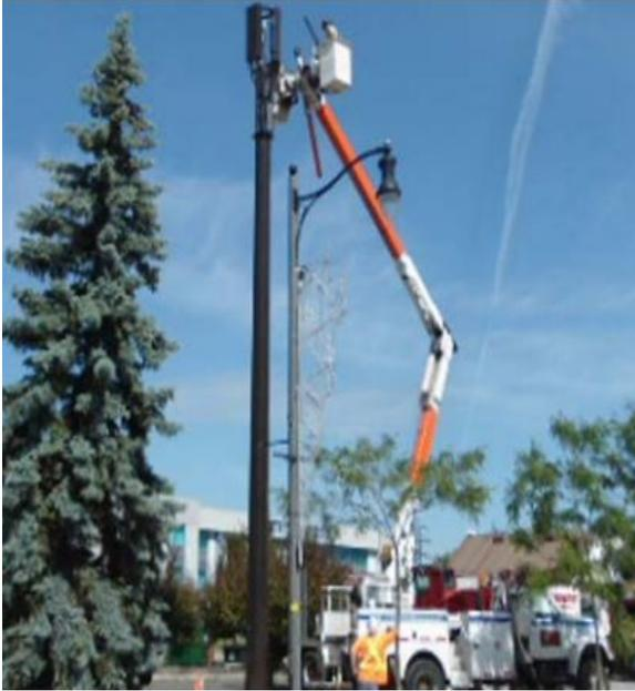
**Exhibit 14.** The location context for this small cell monopole is not reasonable because it creates a cluttered appearance. In addition, the antenna is larger than the diameter of the pole, lacks of pole base of comparable volume, and is vertically out-of-scale to the existing streetlights.
