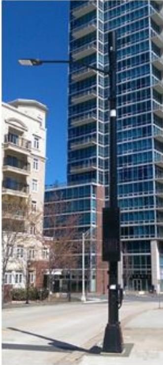
**Exhibit 4.** The antenna, by Valmont, is painted black to blend-in with the pole and is in scale with the pole base. The arm is within the top 15-20% of the pole height, appearing in balance. This may be an acceptable design depending on the location context and color, which should be consistent with existing poles in the immediate vicinity.
